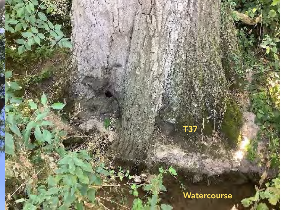
IMAGE 3: A view looking south at the root-collar of T37 showing the close proximity of the watercourse and the witness marks of high water.
